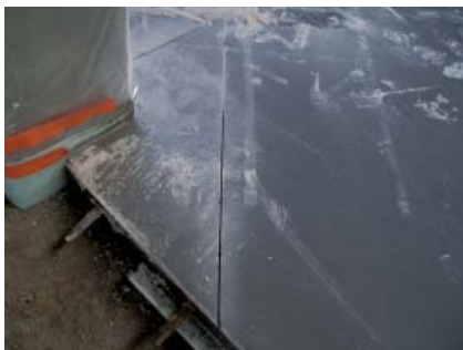
Detail HALFEN Load joint in the column area. NIKE sales center in Laakdal, Belgium.
