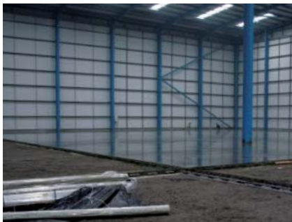
HALFEN Load joint for defining daily sections. TWINTEC logistics building in Liverpool.
