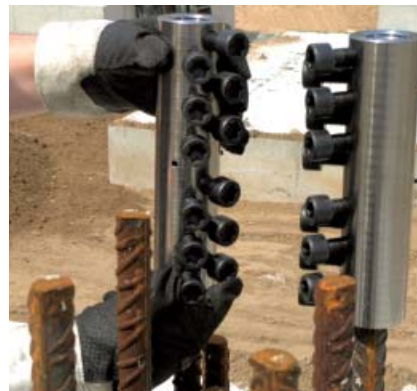
HGC Grip Connector during installation
